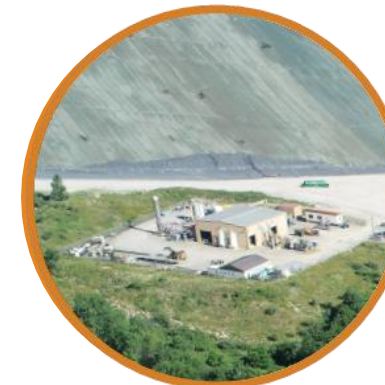
Landfill with Gas Recovery
