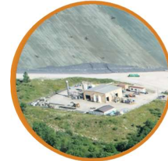
Landfill with Gas Recovery
